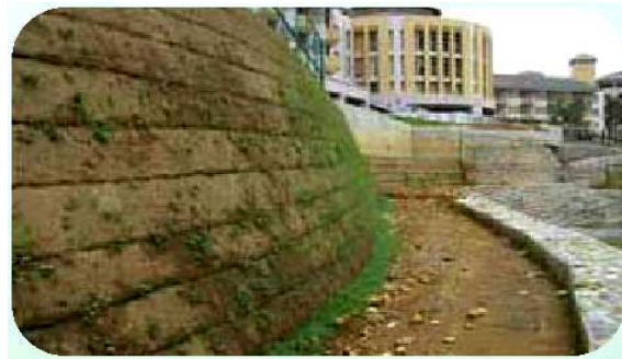
Athletic Field Landscape Construction in Pu-Tai Elementary School Project
