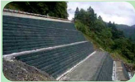
Yilan First Road Roadbed Repair Construction Project
