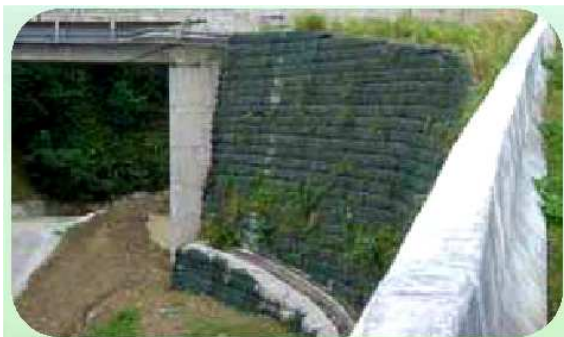
Abutment Construction in Tamkang University Lanyang Campus
