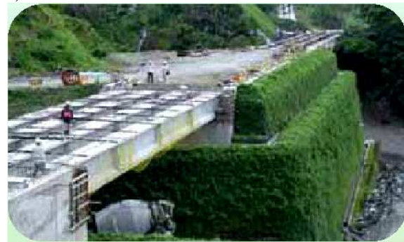
Abutment Construction in Yuchang Highway Building Project
