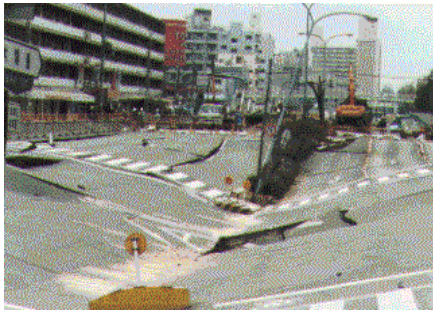
Figure 3. The effects of liquefaction in Kobe city area (© www.seismo.unr.edu/ftp/pub/louie/class/100/effects-kobe.html )
